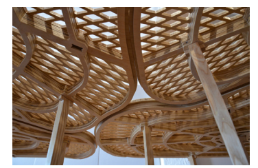
UNDERSIDE All of the design development of this project is located on the underside of this table, much more closely resembling a structural frame model. With 30 individual legs plugging into 6 separate frames, the table had to be mocked up iteratively to test the stability of such designs as material artifacts. We wanted to control the design detailing and not resort to steel, eventually thickening the underside in certain locations and allowing it to remain thin in others. Softening a standard table shape to reflect the distortions of material present in Thonet's original chair produced a design which was also much more unpredictable, requiring the combination of design and build to test our designs for material quality marking an exchange between design and fabrication. In the end not only is the shape distorted but the sequence of design to production is also distorted as the process produced feedback between materials and representation, iteratively distorting itself.
